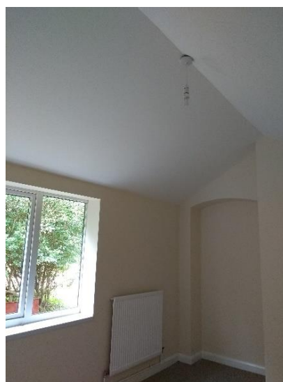
Following works required by enforcement notice
